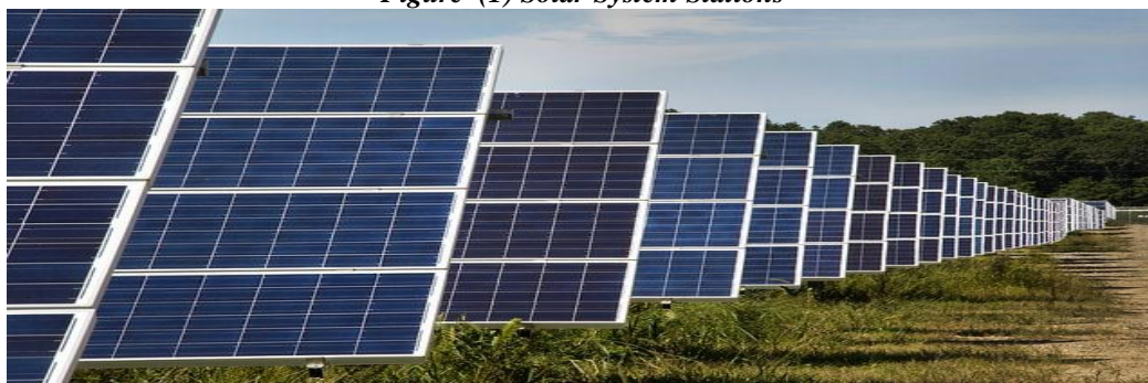
Figure (1) Solar System Stations
